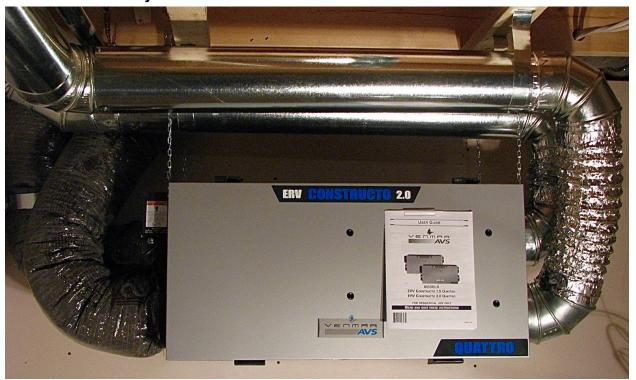
A heat recovery ventilation system (HRV) transfers heat between the old exhaust air and new fresh air. The air streams never mix during this process. Because an HRV effectively transfers heat, the system also helps keep heating costs low. An HRV is often recommended for colder climates.
